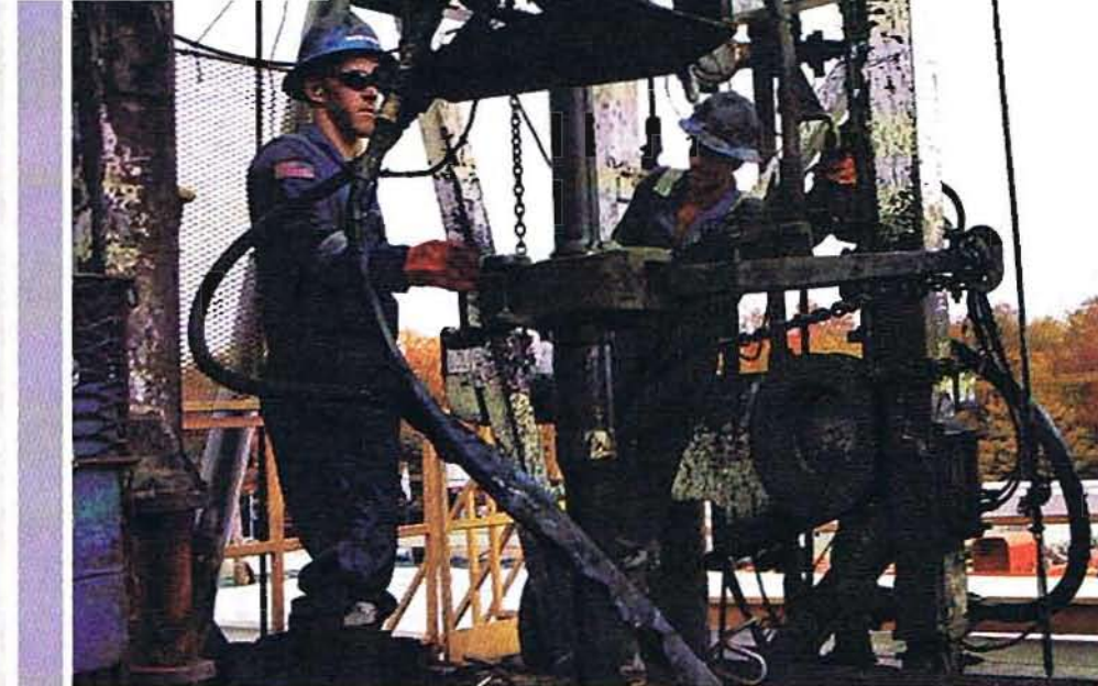
Workers remove pipe from a gas well drilled in Bradford County
